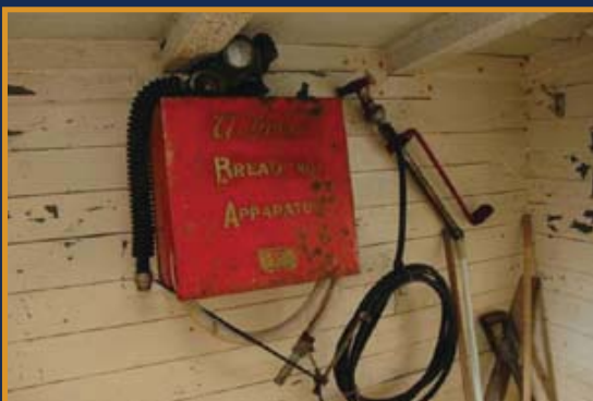
Breathing apparatus and a stirrup pump hanging on the entrance porch wall
