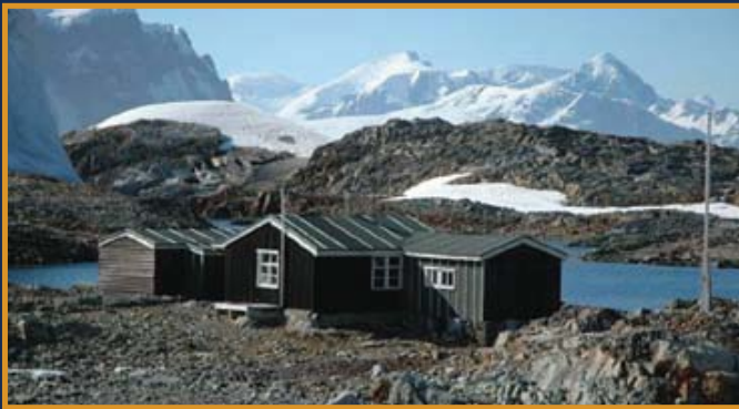
The hut seen from the north and showing the various different builds
