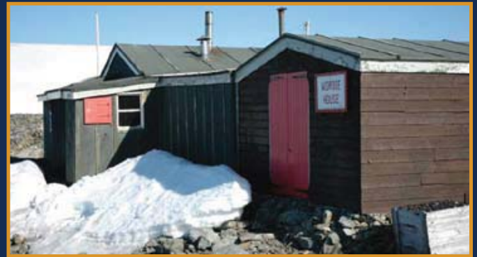
The hut seen from the south showing how close it is built to the sea
